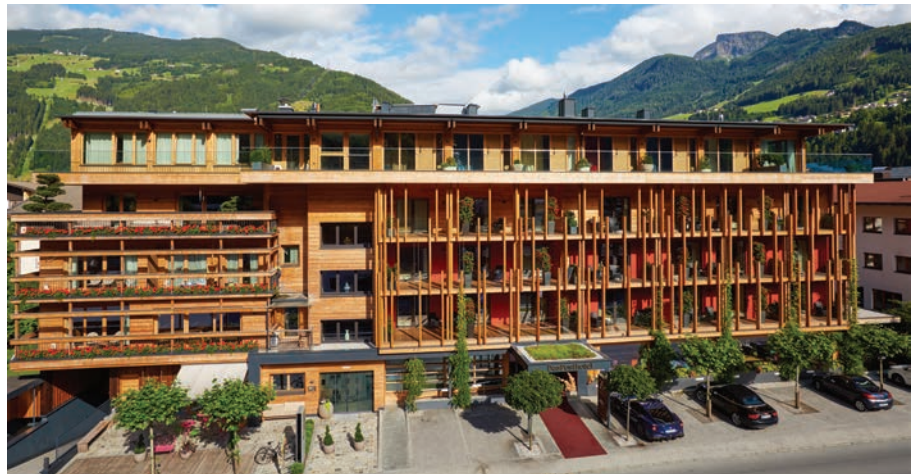
Above left: The Fügen log yard Above right: The Das Posthotel in Zell am Ziller has been extended with CLT
